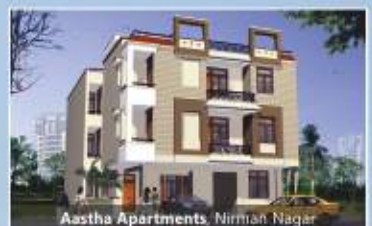
Aastha Apartments, Nirman Nagar
