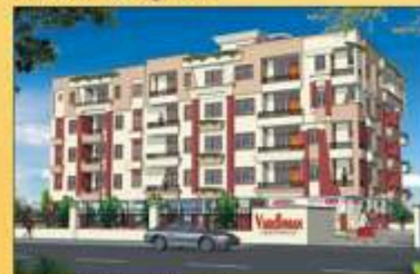
Vardhman Apartments, Bonipark
